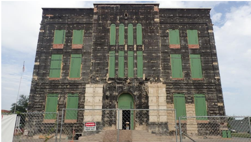
Figure 2. Current appearance after removal of non-historic stone overladding.
