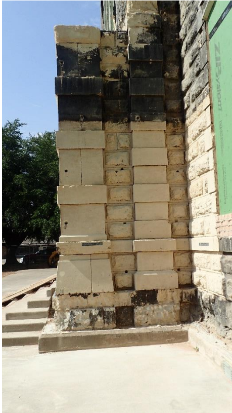
Figure 21. Prosoco Limestone Restorer, Reclaim, and Afterwash: majority of coating removed: Trial 21.
