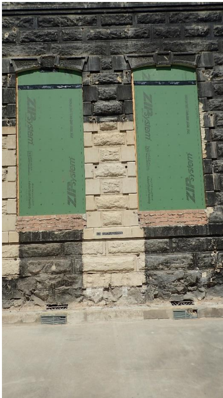
Figure 14. Prosoco Fast Acting Stripper, Limestone Restorer, Reclaim and Afterwash: Trial 16.
