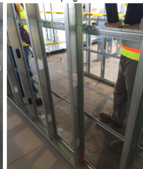
Telescoping Metal Studs
