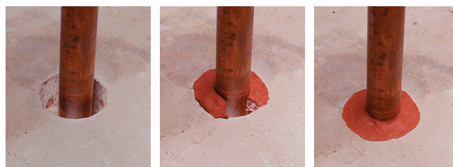
Through-penetration being firestopped.
