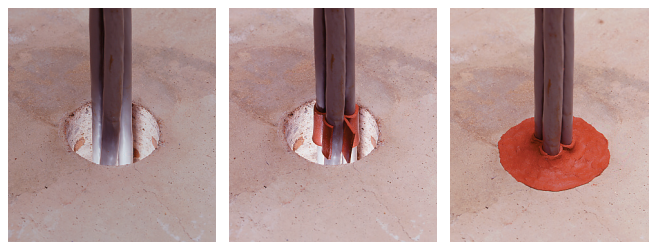
Cable bundle being firestopped.
