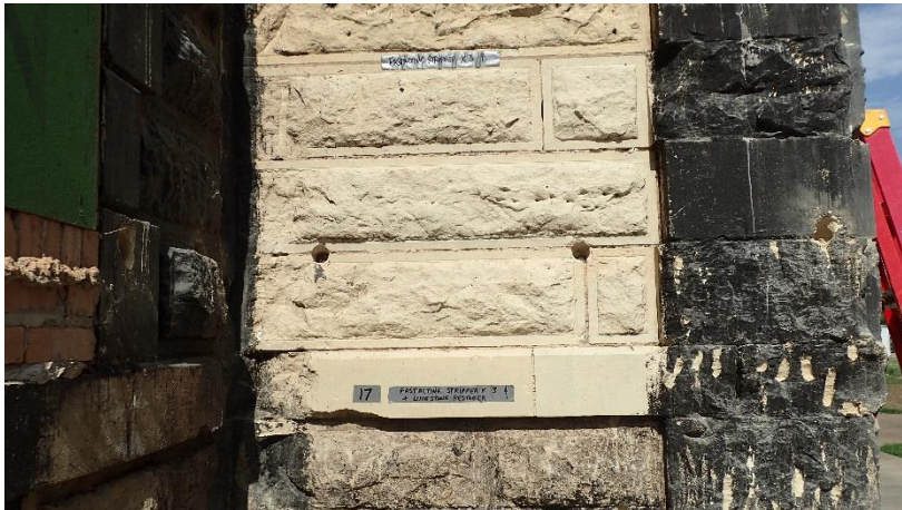
Figure 16. Prosoco Fast Acting Stripper and Limestone Restorer: majority of coating removed: Trial 17.
