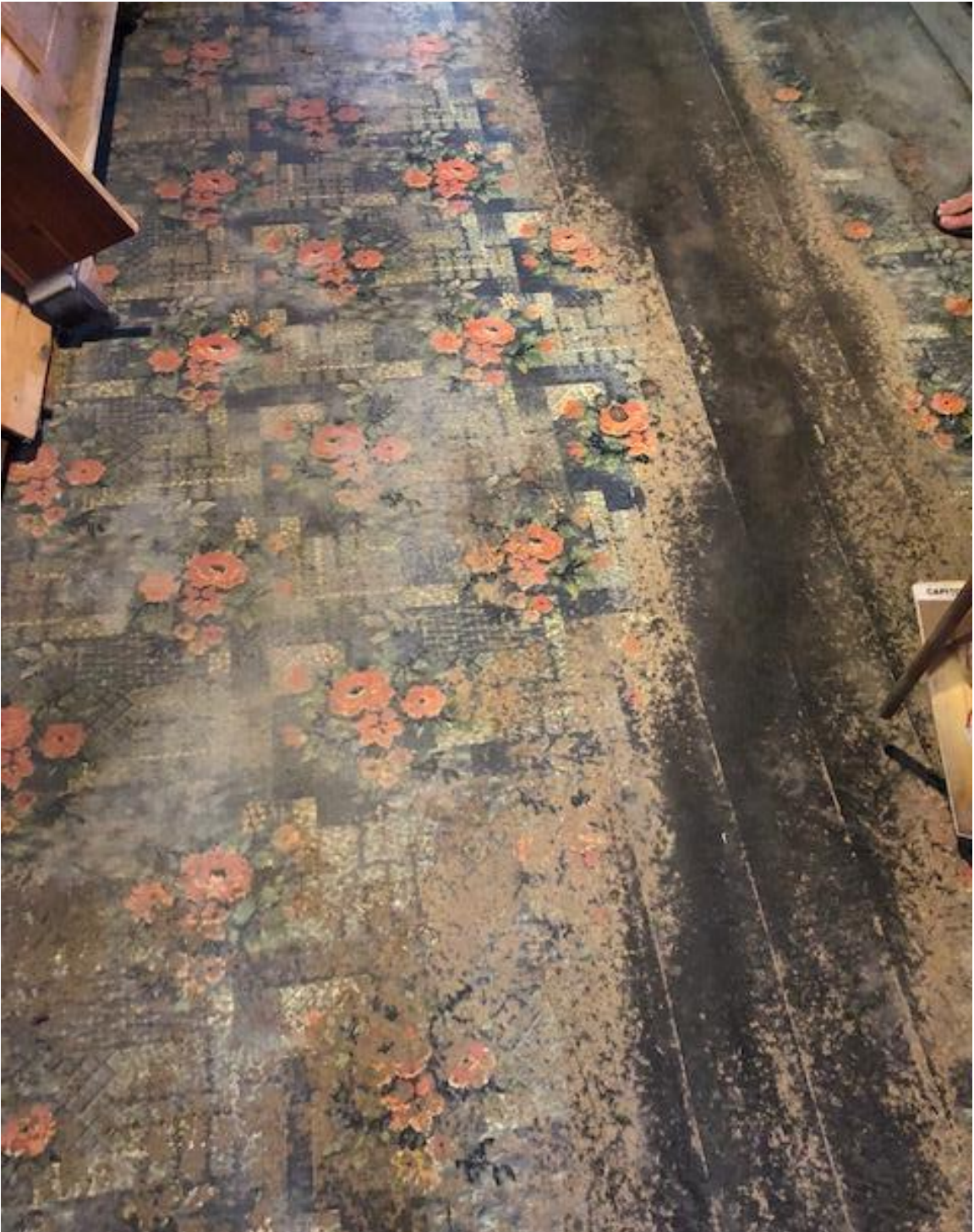
Close-up of previous wall to wall installation. Note how the product is wearing away into the wood.
