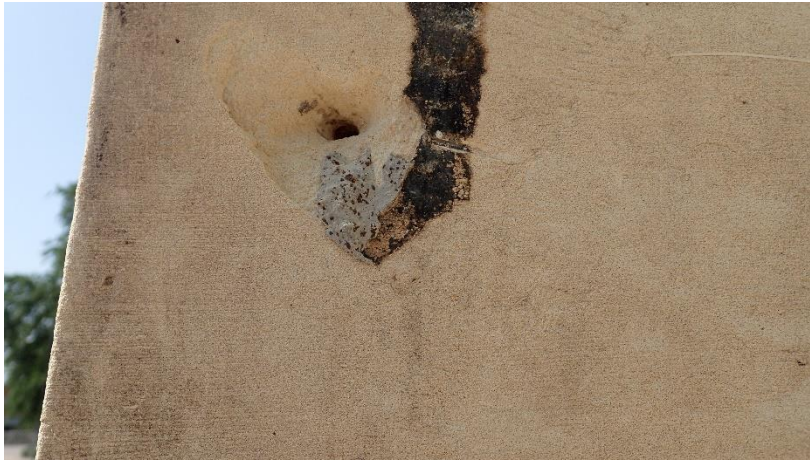
Figure 8. Grey grout from the anchors and red surface corrosion.
