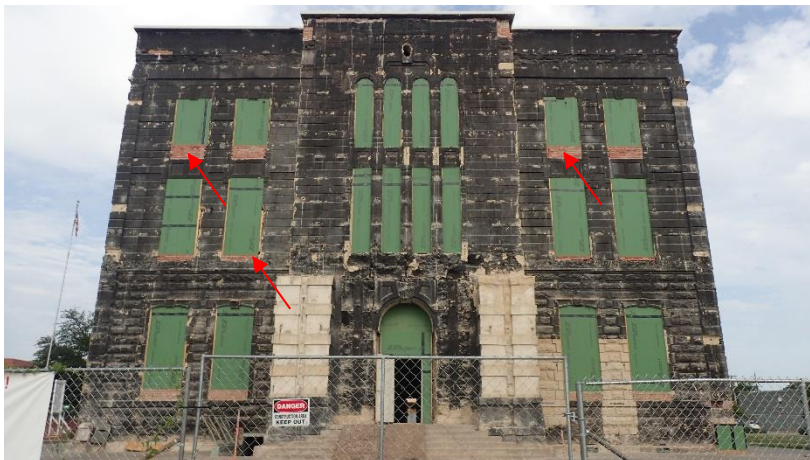
Figure 10. Areas of brick infill marked with red arrows.
